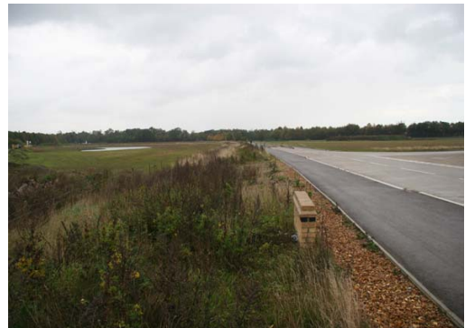
10 - Guided Bus Route - Large Orchard
